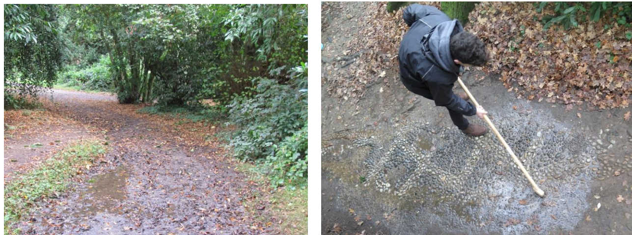
Left - existing paths in poor condition. Right - HCC conservation team uncovering the Shell house Path for survey December 2016.
