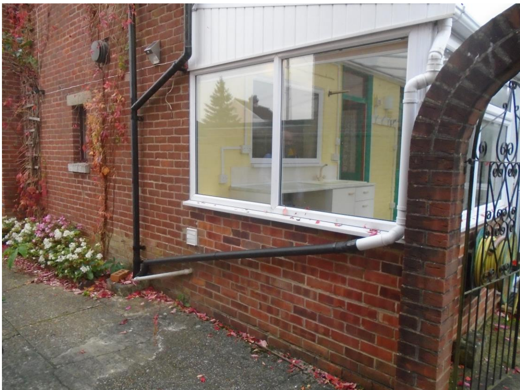
Figure 4. Conservatory to be removed.
