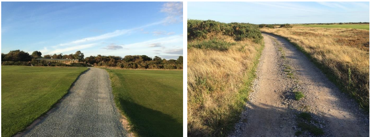
Figure 4 – a) looking north along eastern part of construction route, already laid with hardcore; b) construction track that will receive a hardcore layer.
