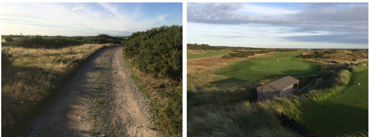
Figure 5 – a) construction track that will receive a hardcore layer; b) general view east from development site across Links.
