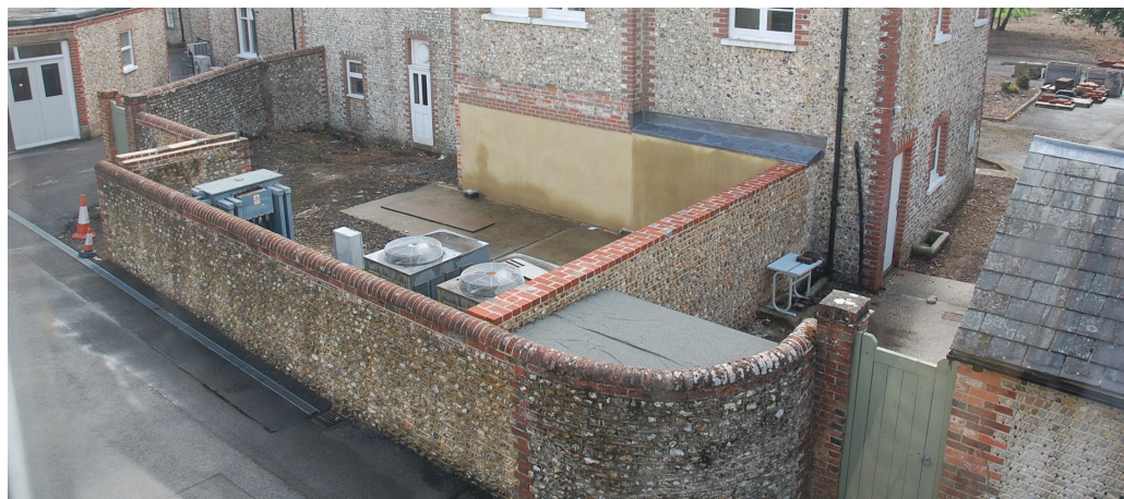
Existing flint wall.
