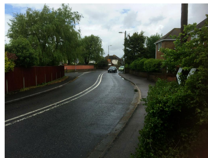
Clear View to the North in excess of 60m to rear car in view provided (note hedging which is on site to be cut back and reduced to allow visibility splay view)
