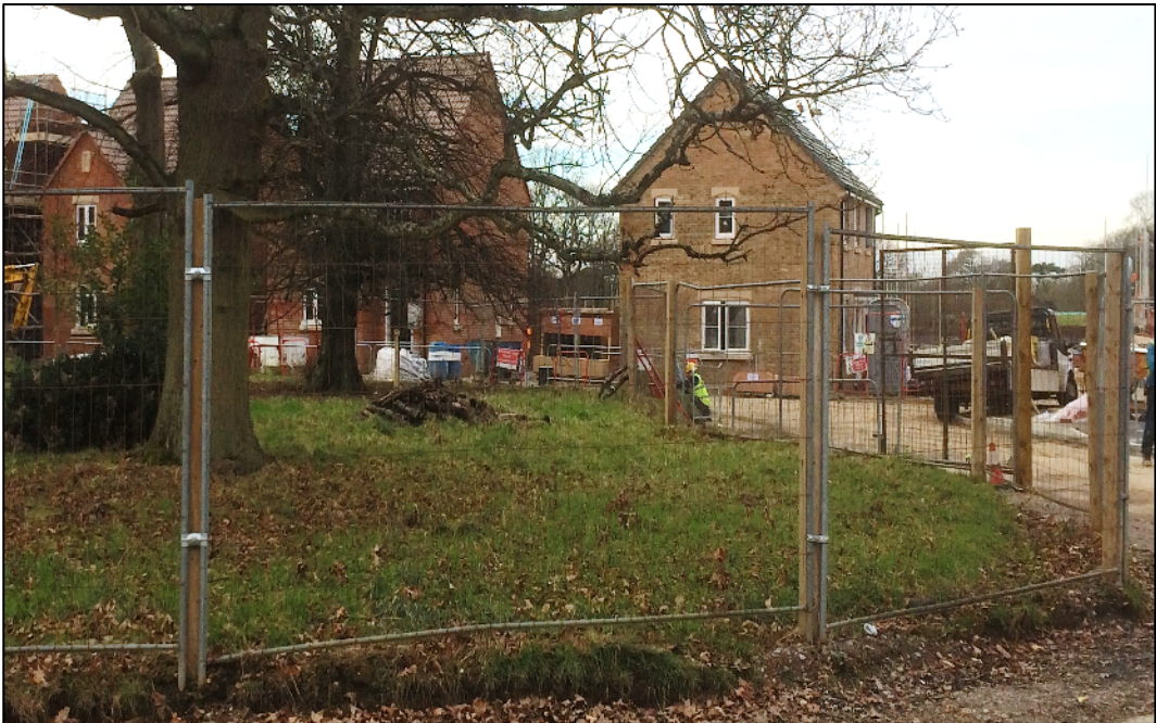
Weld-mesh panels on wooden posts
