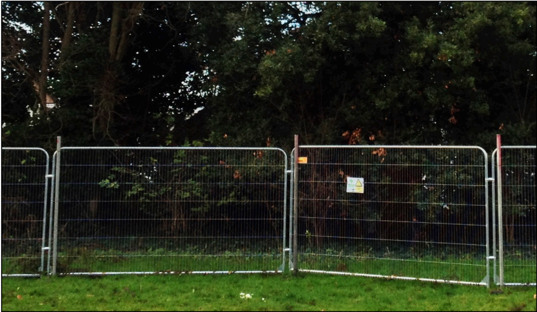
Weld-mesh panels on scaffold uprights
