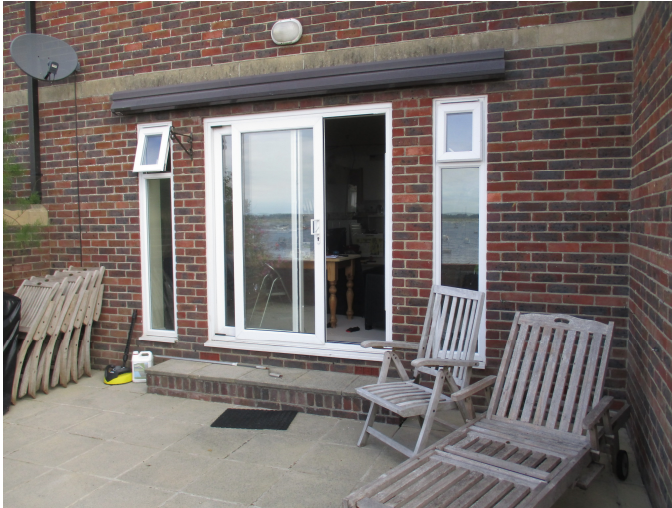
Fig 3 – View of rear patio doors onto the rear terrace
