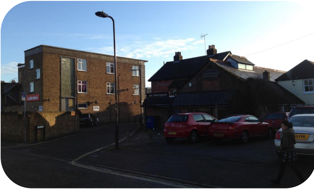
Application site and side of the building at nos. 75-75b London Road, visible from Swiss Road. The area to the rear of the public house is used for servicing and ancillary car parking.
