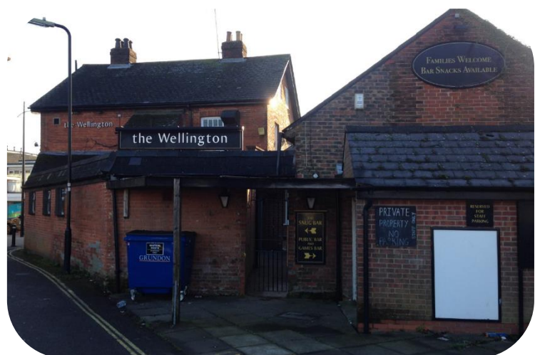
Rear of Former Wellington Public House
