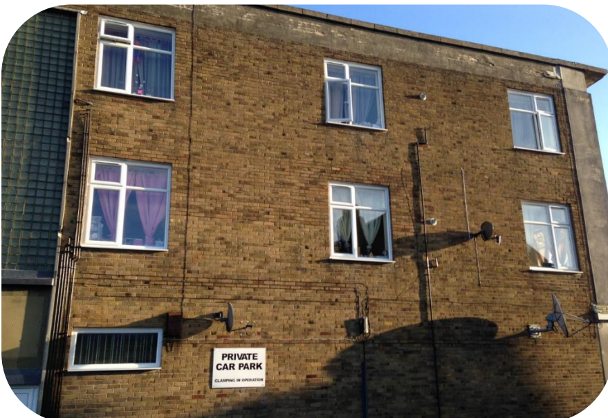
Existing first and second floor windows at the side of nos. 75-75b London Road. The use of the rooms that the windows serve appears to be bedrooms (left and central windows) and a secondary window to the lounge on the right hand side.
