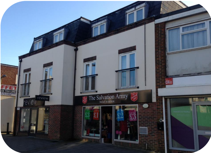
Existing commercial units on the ground floor with 2 storeys of self contained flatted accommodation above, at no. 254 London Road.
