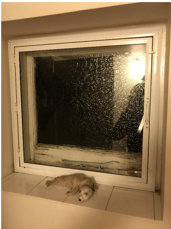
Figure 7: Internal view of window C
