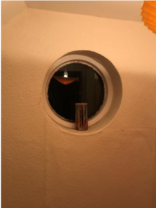
Figure 8: Internal view of window D
