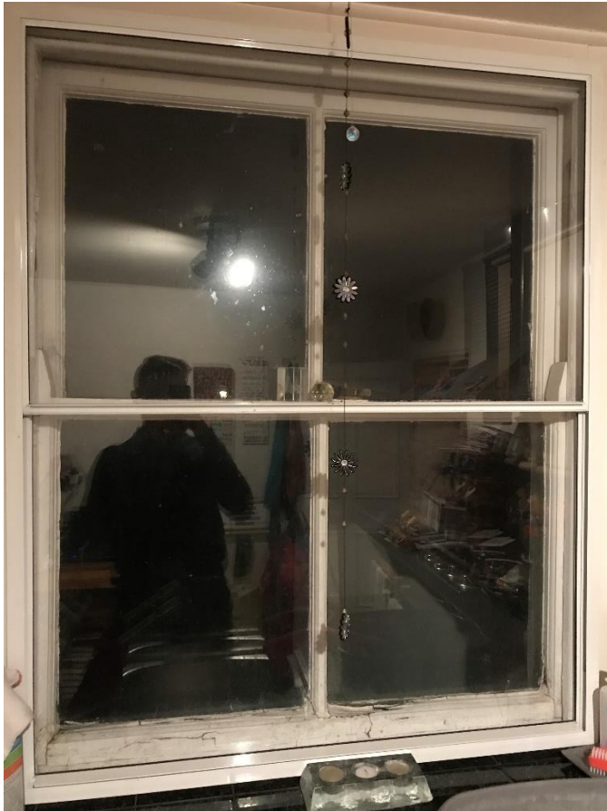
Figure 6: Internal view of window B
