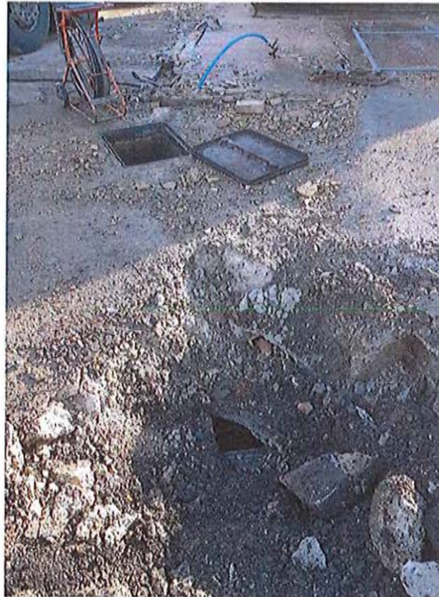
Plate 1. Public FWMH 3902, (broken corner of cover slab in foreground)
