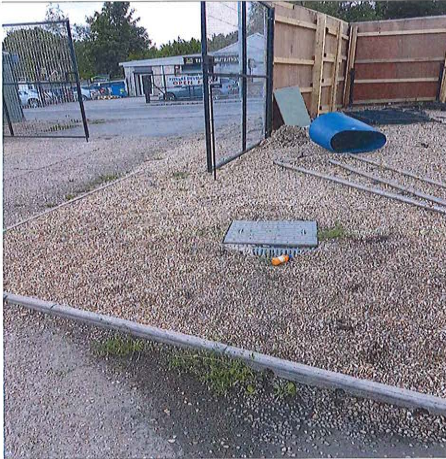
Plate 3, Gravel area next to site entrance found to drain to FWMH 3902 Note holes in path edging to permit drainage from macadam paved area to drain.
