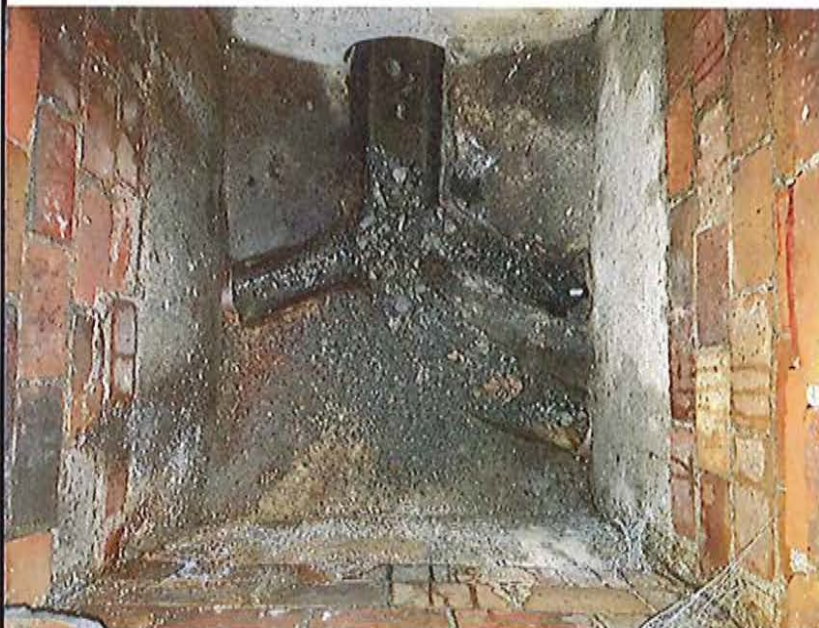
Plate 1. Public FWMH 3902, (broken corner of cover slab in foreground)
