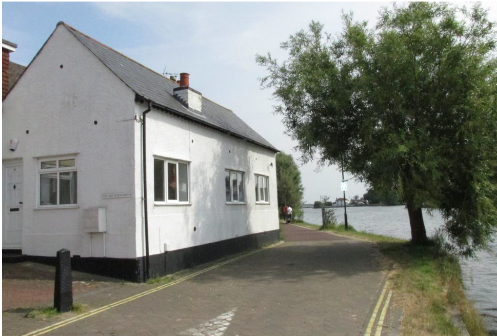
Water fronting elevation of the dwelling.
