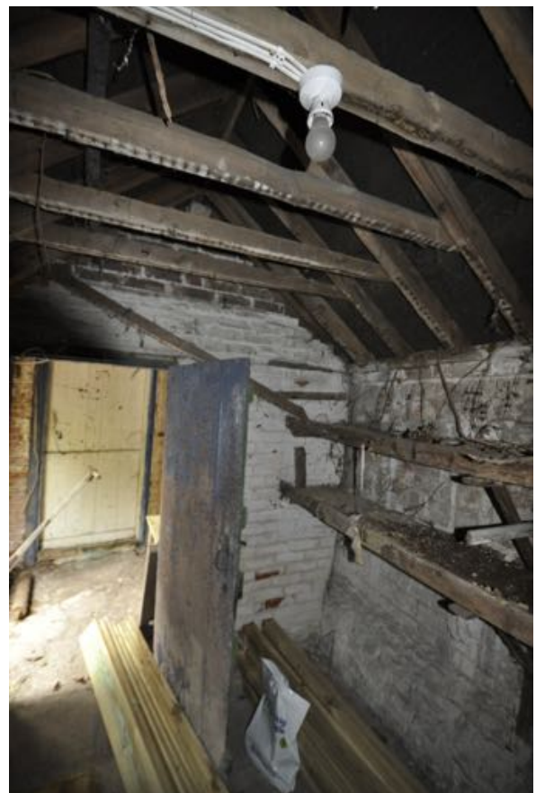
Potting sheds internal
