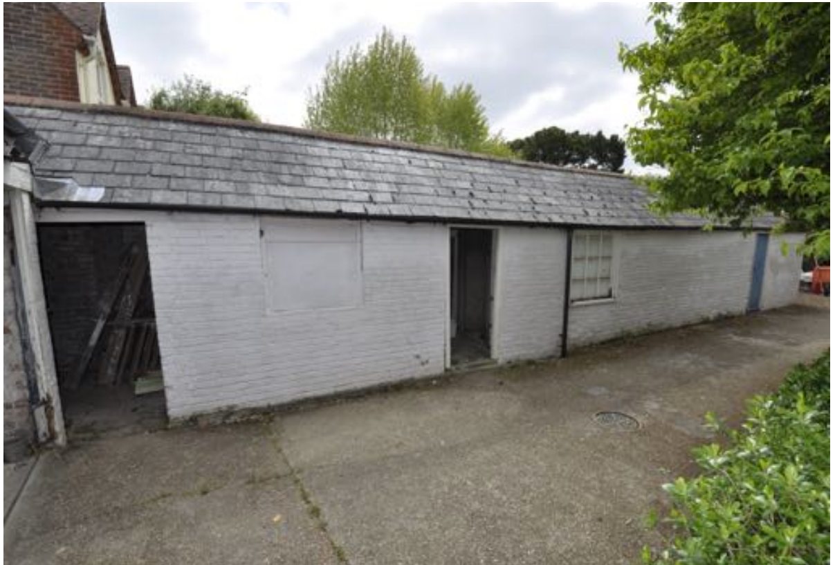
Potting shed - West elevation view
