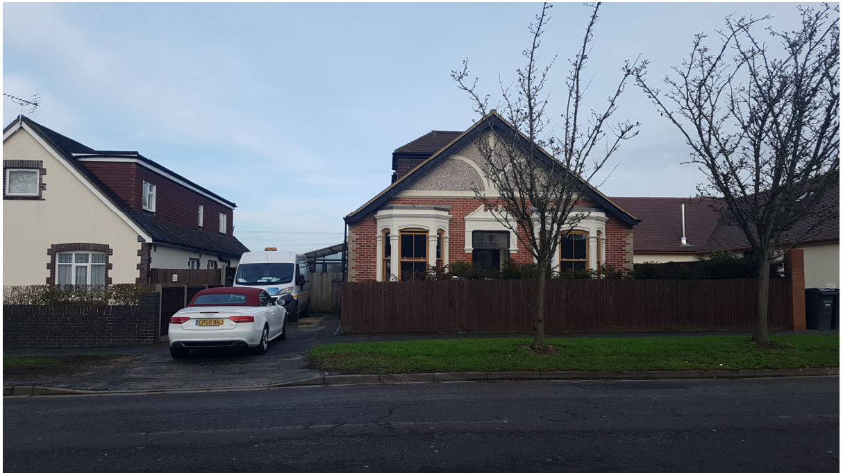
View of the main elevation.
