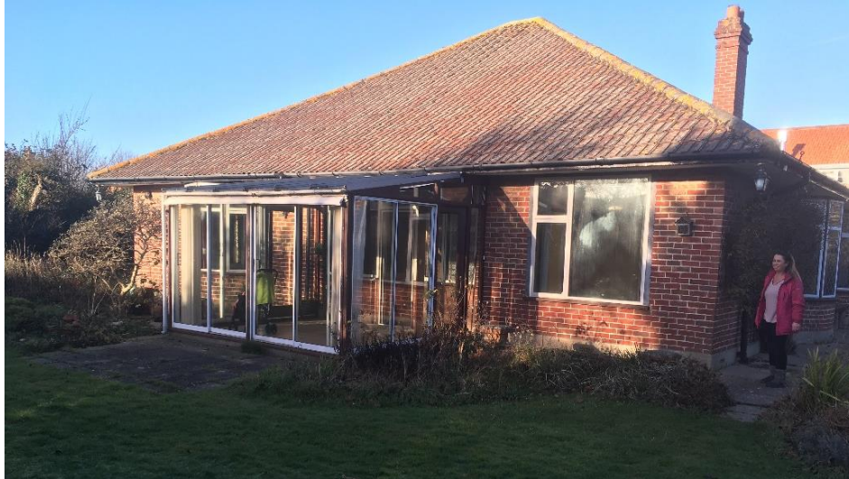
Side of the property from the garden showing existing conservatory (main house entrance)
