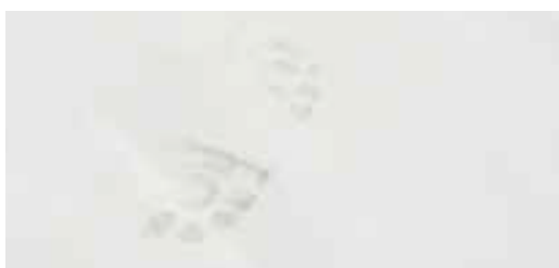
Dirty footprint caused by installation
