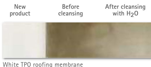
White TPO roofing membrane
