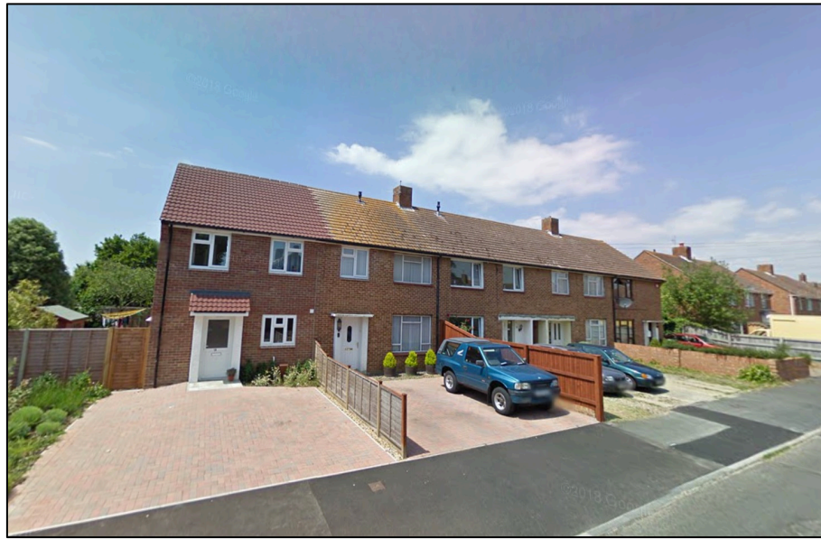
Figure 3: Narrow terraced house on the southern end of Ilex Walk, close to the appeal site
