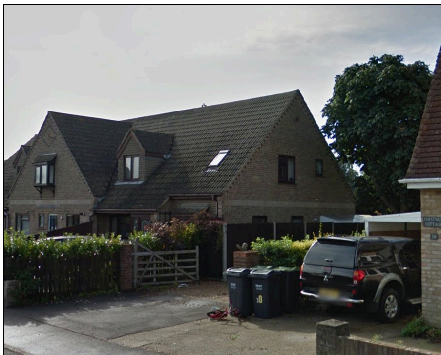
Figure 5: Image of the side windows in the neighbouring property at number 32a
