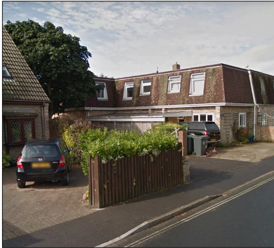
Figure 6: Image of the side windows in number 30
