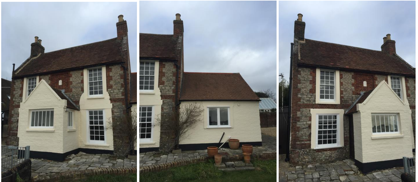
Front Elevations prior to restoration work in 2015
