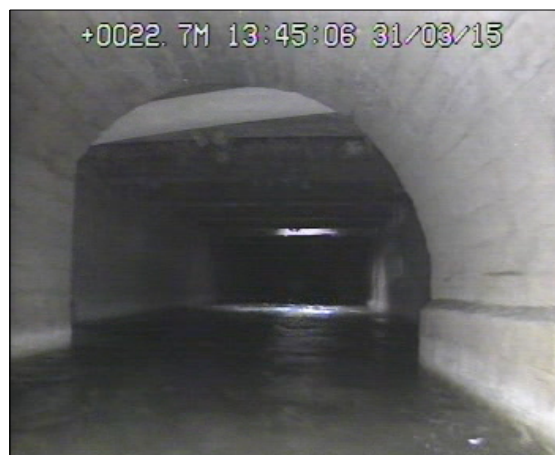
Photo: 3_13A, 00:04:53 22.7m, Shape changes to arched, 1500mm high, 1700mm wide
