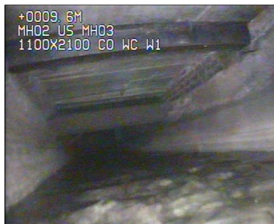
Photo: 3_6A, 00:01:53 9.6m, Line deviates left
