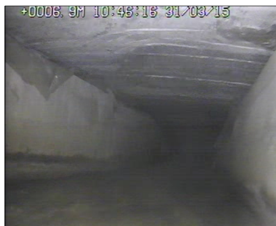
Photo: 1_7A, 00:02:15 6.8m, Material of drain/sewer changes to Concrete
