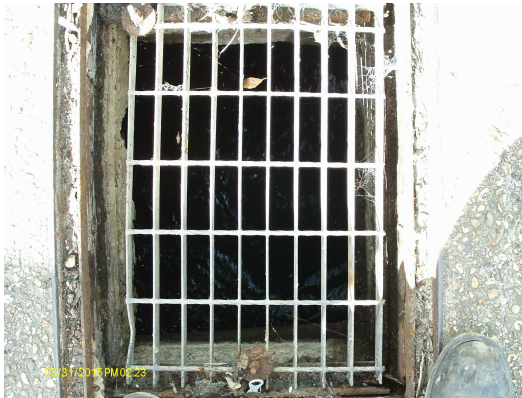
View into MH03
