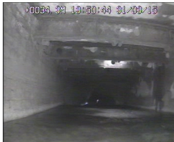
Photo: 3_14A, 00:10:30 34.3m, General remark Remarks: MANHOLE WITHIN VIEW APPROXIMATELY 3M AWAY
