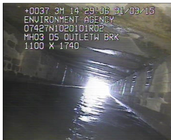
Photo: 4_9A, 00:04:03 37.3m, Shape changes to rectangular, 1000mm high, 1630mm wide
