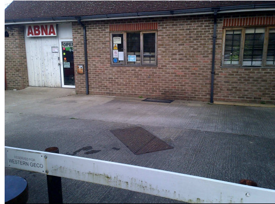
MH01 location outside Units 15 & 16 of the Old Flour Mill
