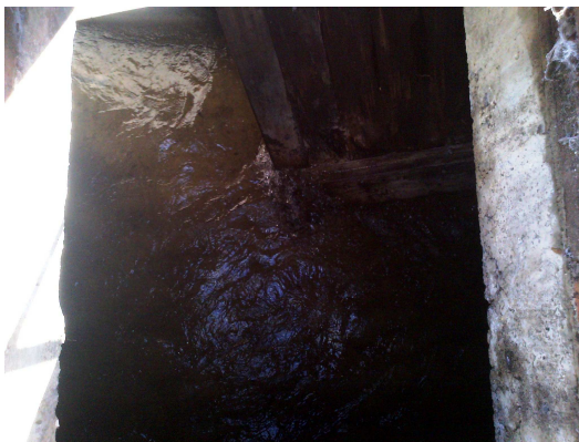
View into MH01
