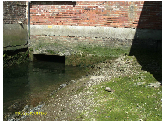
View of the Outlet located on the South side of No.8 Chequers Quay on the South side of Queen Street
