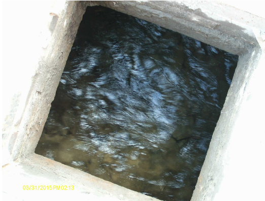
View into MH02
