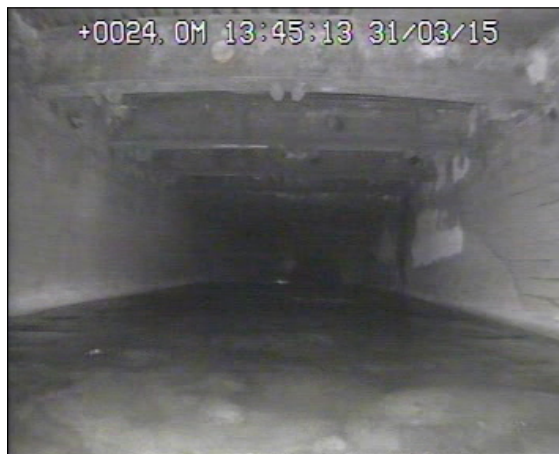
Photo: 3_14A, 00:00:05 24m, Shape changes to rectangular, 1140mm high, 1700mm wide
