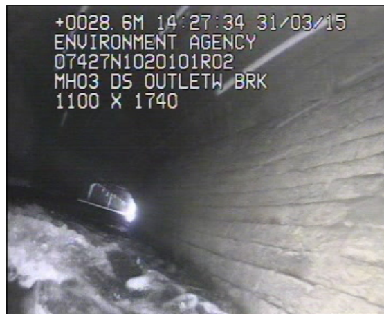
Photo: 4_8A, 00:02:31 28.6m, Line deviates left
