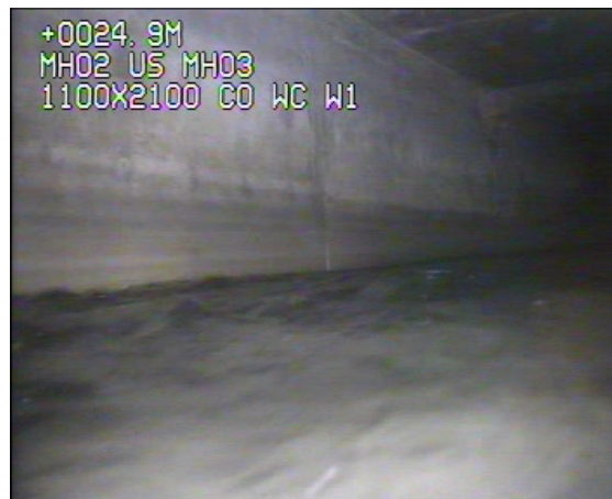
Photo: 3_9A, 00:04:07 24.9m, Line deviates right
