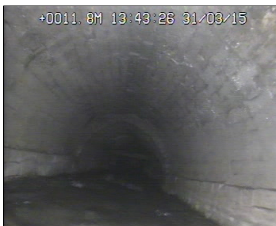
Photo: 3_3A, 00:03:12 11.8m, Dimension changes, 1400mm high, 1500mm wide
