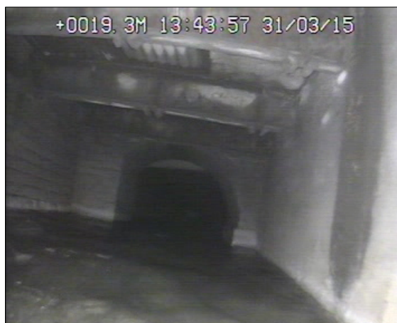
Photo: 3_11A, 00:03:43 19.3m, Dimension changes, 2000mm high, 2000mm wide Remarks: SQUARE SHAPE
