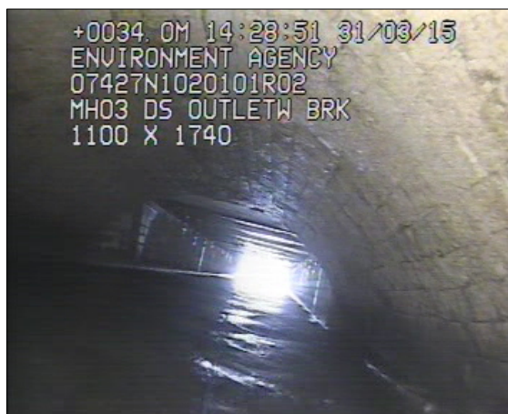
Photo: 4_9A, 00:03:48 34m, Shape changes to arched, 1000mm high, 1400mm wide Remarks: APPROXIMATE SIZE
