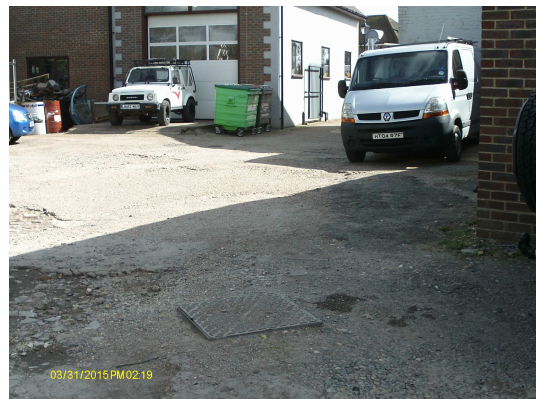
MH02 location at the rear of Lilywhite Bros Ltd garage on Queen Street
