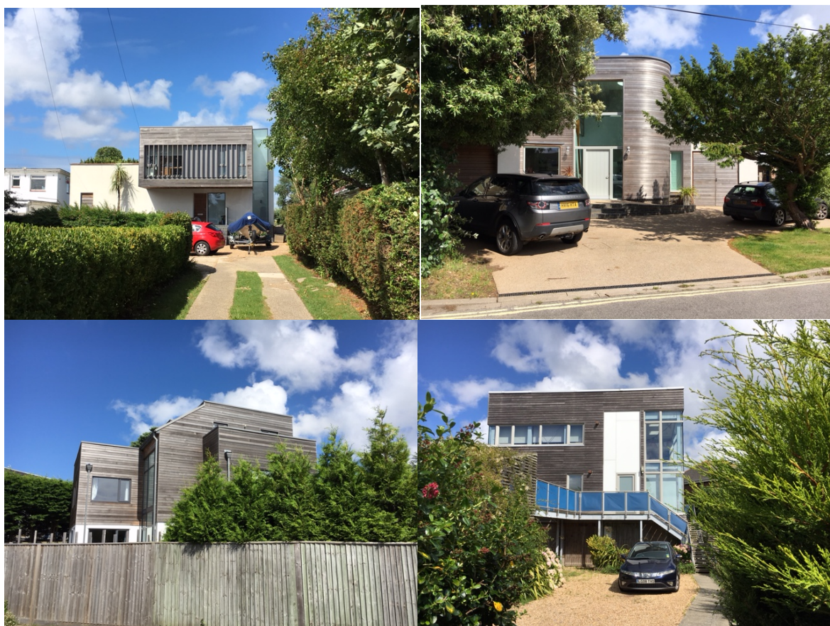
Local examples where wood cladding is used in more recently constructed homes
