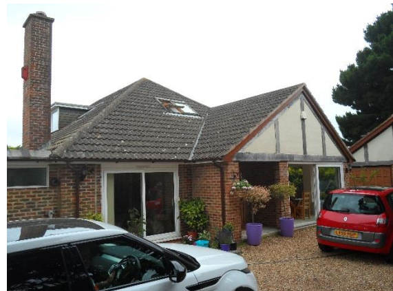
View of west elevation entrance with hipped main roof and high level 'velux' roof windows.
