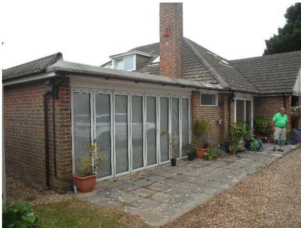
View of entrance area on north elevation
