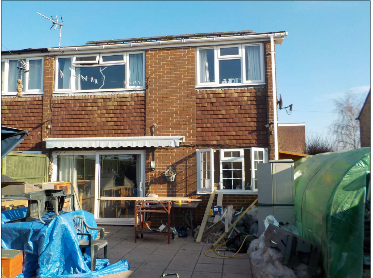
Rear of No. 14A Gordon Road
