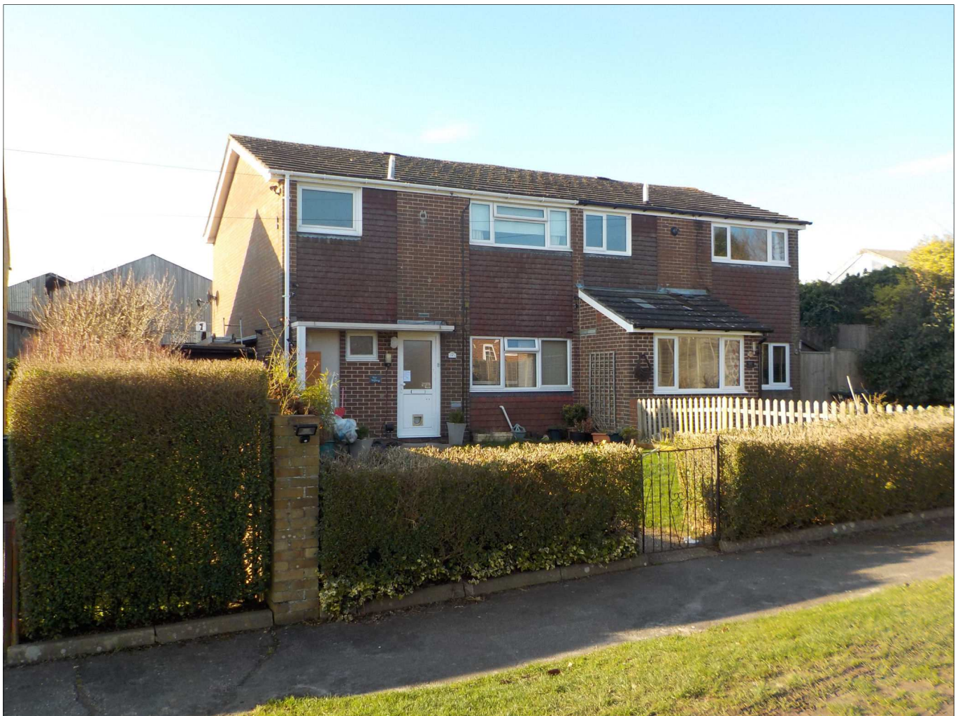
Front of No. 14A Gordon Road
