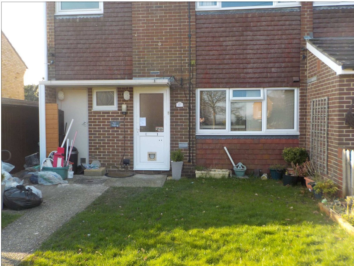
Front of No. 14A Gordon Road
