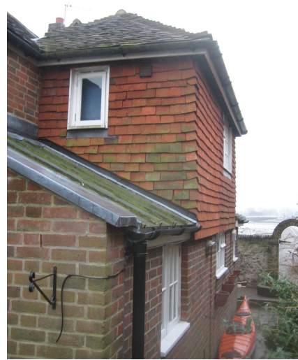
Fig 4 – View looking along the side of the property from the rear, towards the front
