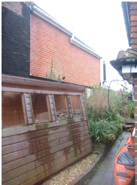
Fig 5 – View looking along the side of the property from the front, towards the rear of the neighbouring property to the west
