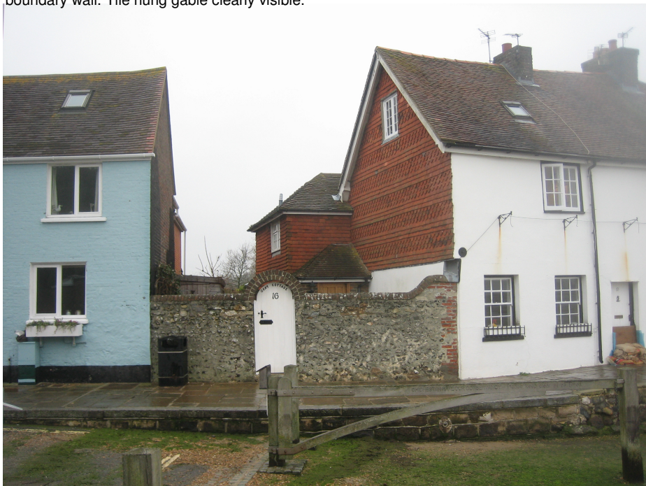
Fig 2 – View of property with entrance door just visible above the top of the flint wall. Existing tile hung side extension visible.
