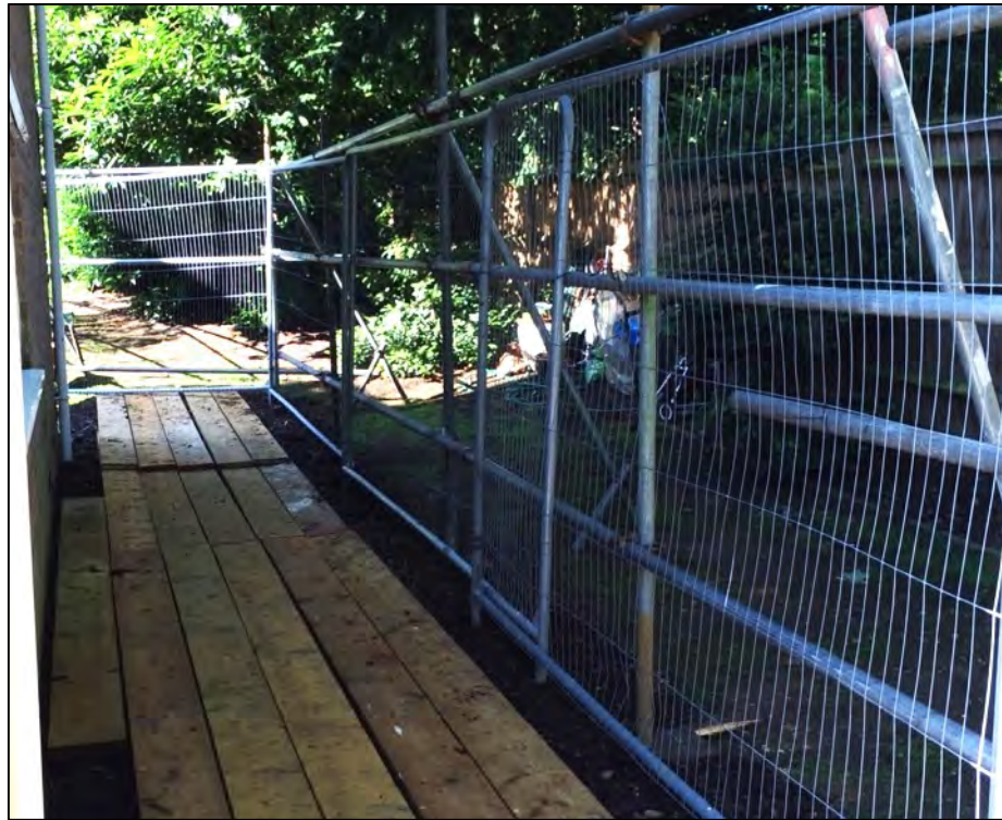
Scaffold board pedestrian ground protection
