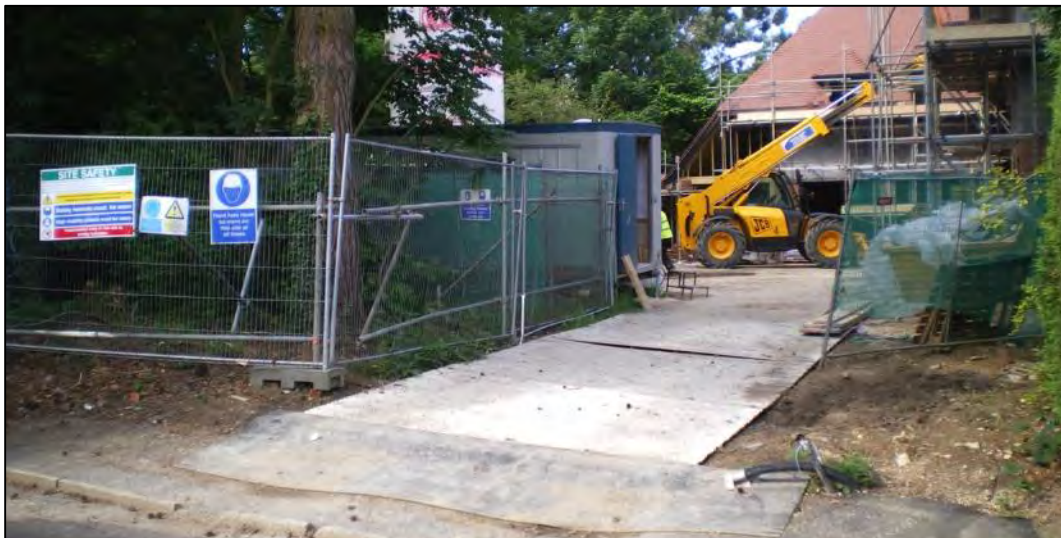
Vehicular ground protection trackway
