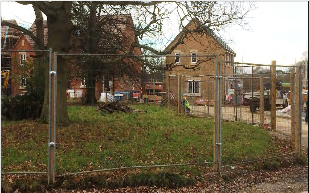
Weld-mesh panels on wooden posts
