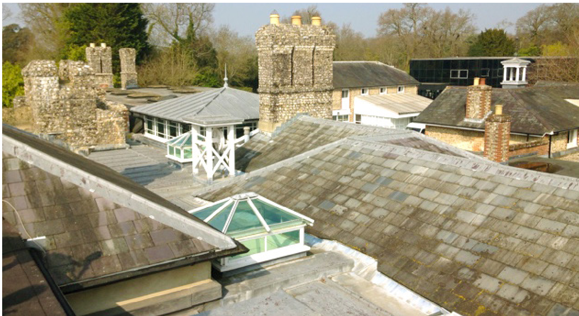
Roofline looking north from the main house
