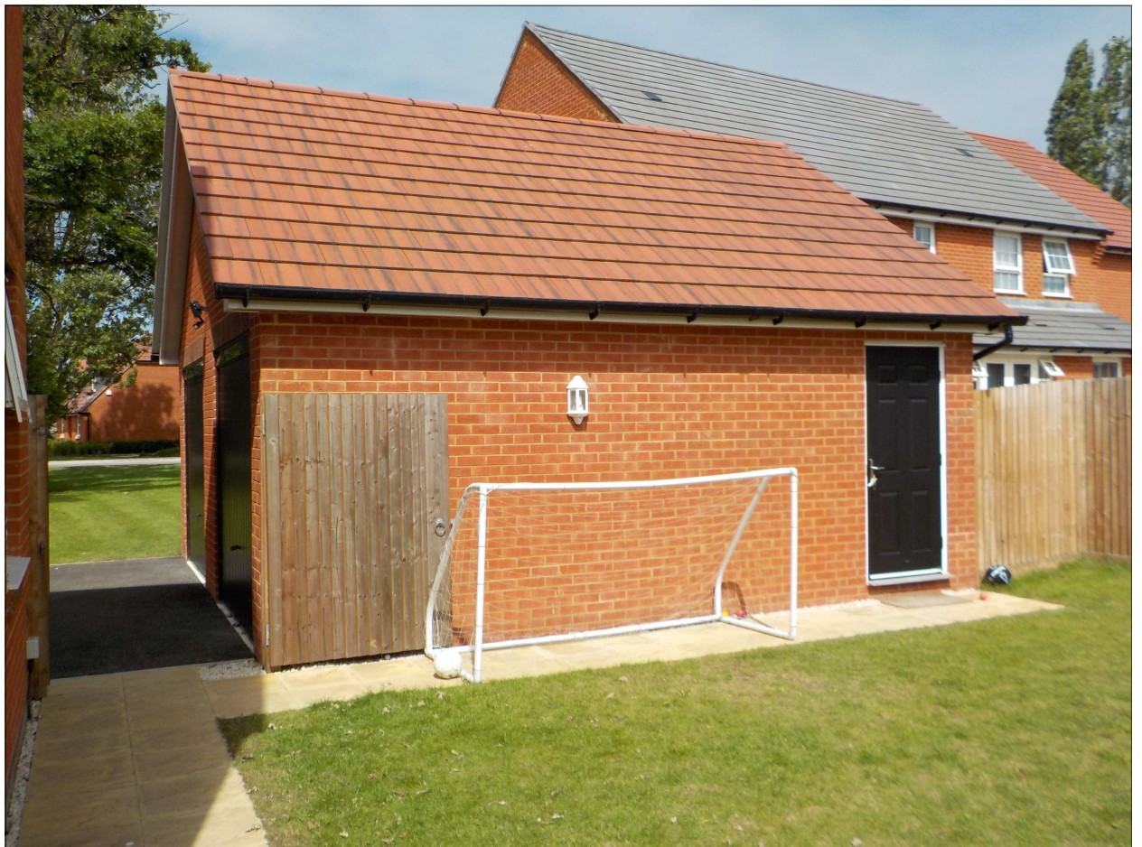
Side views of garage
