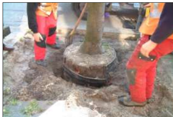
Soil cell image 4: This excavated tree shows the root deflectors that were installed when it was planted seven years previously. The product has deflected roots downwards and prevented damage to the adjacent surfacing. Note that this is a permeable sandy soil and the roots were able to grow beneath the bottom of the deflectors.
