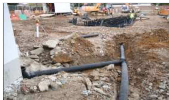
Soil cell image 2: Drainage from adjacent buildings can be directed into Silva Cells, significantly buffering rainwater runoff from urbanised areas.
