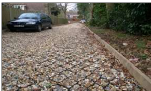
New surfacing image 6: Wooden board pinned in place or held in position with backfilled topsoil can provide more informal and rustic surface edging.
