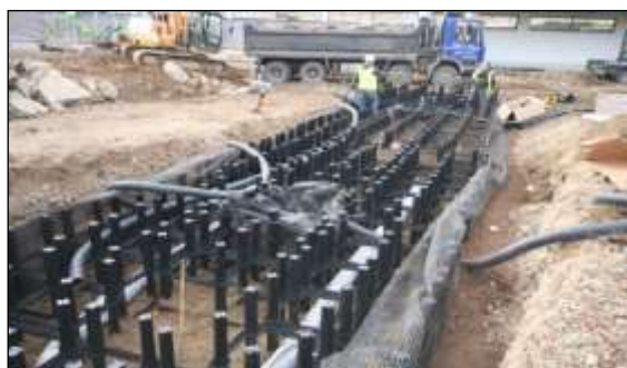
Soil cell image 1: The individual Silva Cells can be assembled in layers and service ducting threaded through before filling with soil and fitting the reinforced tops.
