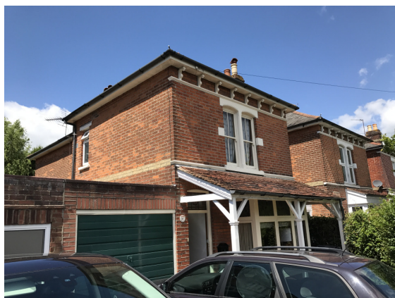
East Elevation displaying front porch and sash windows
