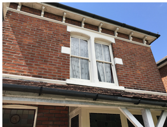
North elevation displaying sash windows in more detail.
