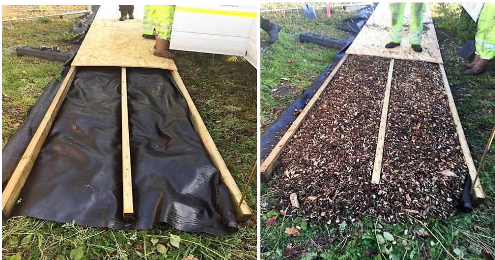
Figure 8. Plywood sheeting used as ground protection.
