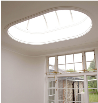
Rooflight over stairs
