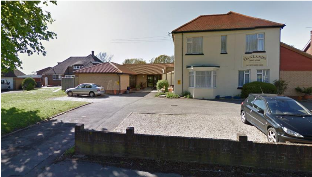
Fig. 5: View from Stakes Hill Road. (Google Streetview)
