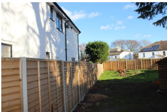
Fig 9: Boundary of site with 48 Station Road (6ft close boarded timber fence)
