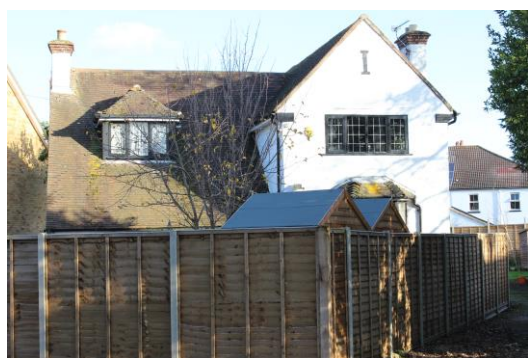
Fig 3: 48 Station Road (front elevation)
