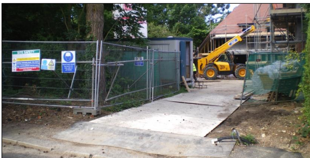
Vehicular ground protection trackway
