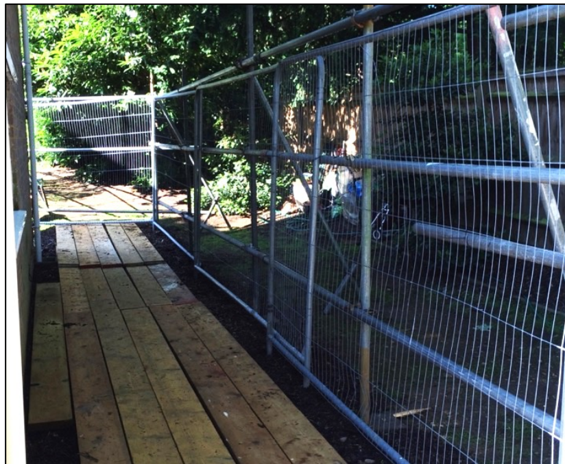
Scaffold board pedestrian ground protection
