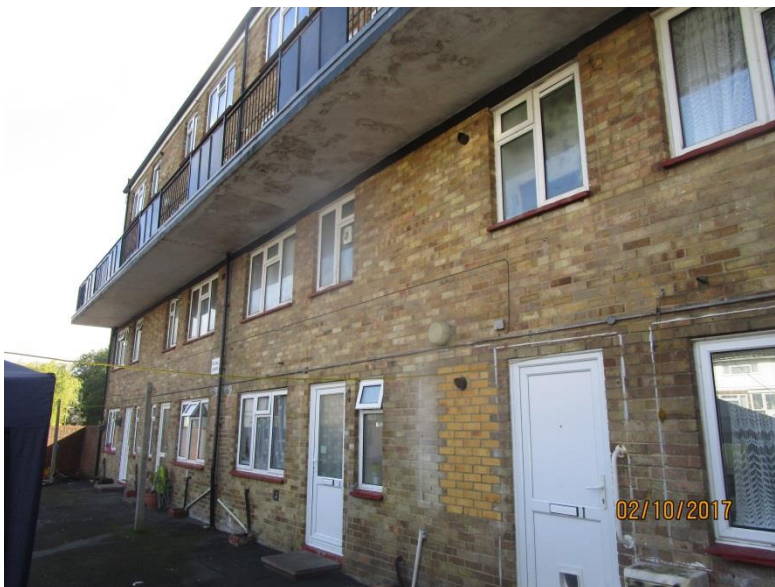
Photo 3 - Rear elevation showing balcony walkway
