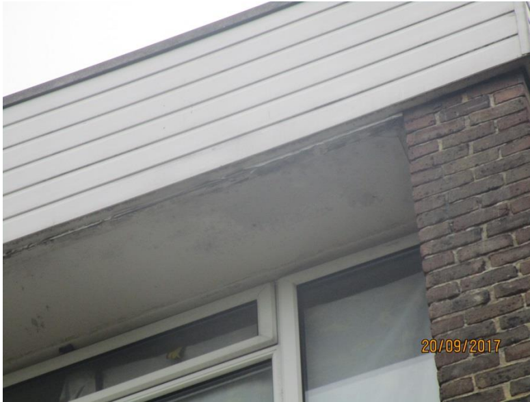
Photo 4 - Existing Fascia Board and Soffit
