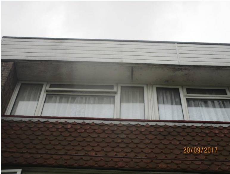
Photo 3 - Existing Facia Board and Soffit
