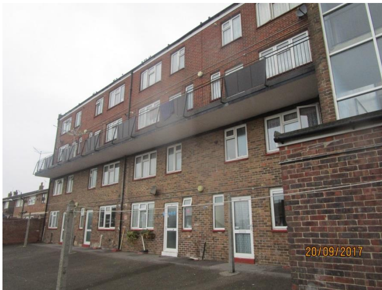
Photo 2 - Rear elevation showing balcony walkway
