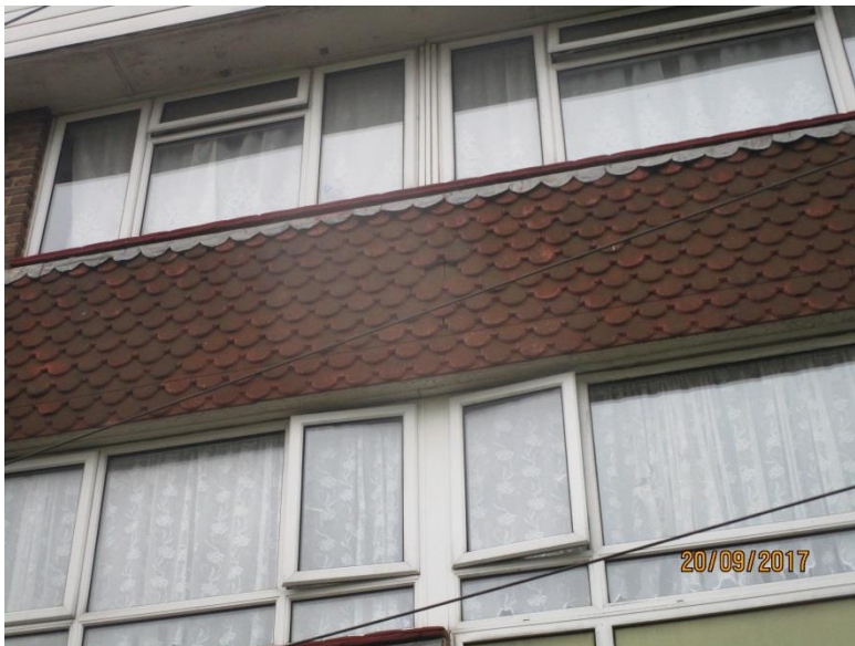
Photo 4 - Tile hanging to front elevation
