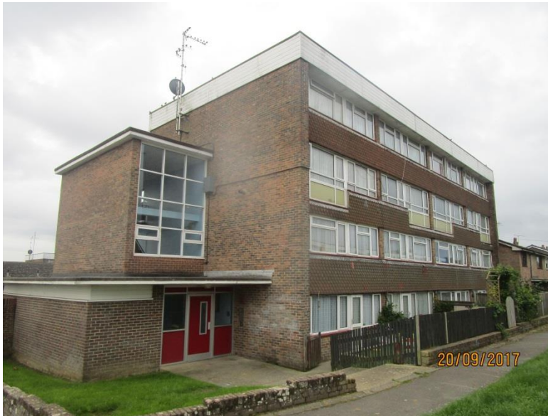
Photo 1 - Front Elevation showing boundary fencing
