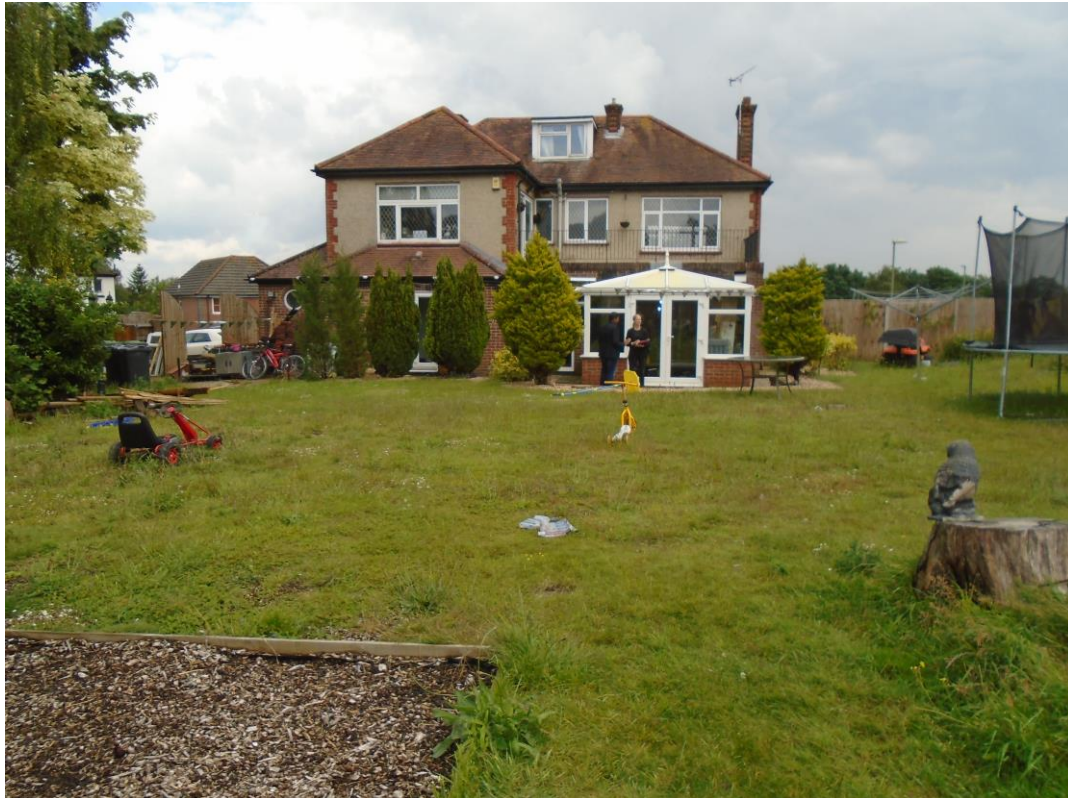
Figure 2. The existing rear elevation and substantial garden area.
