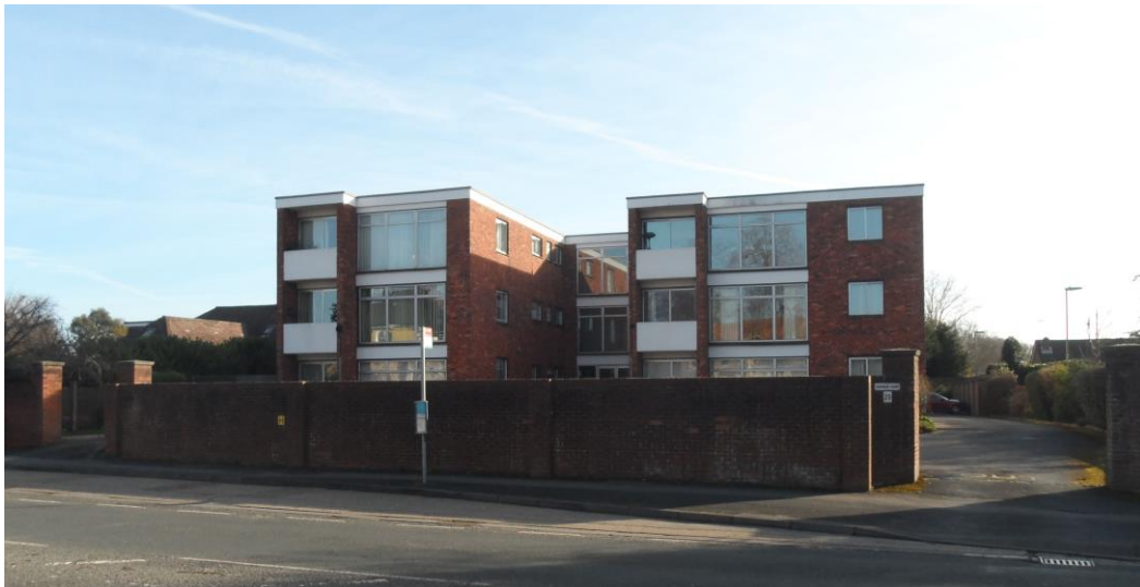
No 29 Langstone Road, Langmead Court, Large 3 storey block of Flats
