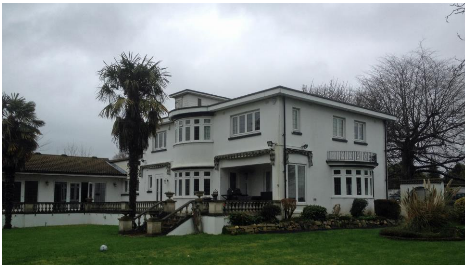
Existing flat roof has a collection of redundant chimney stacks, vents and a water tower
