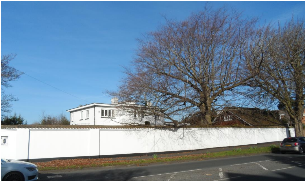
View of property boundary wall to the 'White House' obscuring the ground floor with the trees semi-screening the upper floor. When viewed from further north the garage roof substantially screens the upper floor of the main house in all seasons.
