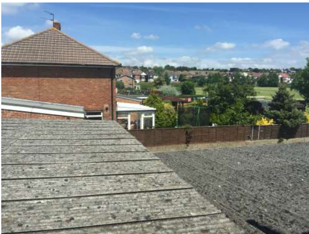
View towards 19 Westways from existing hall window
