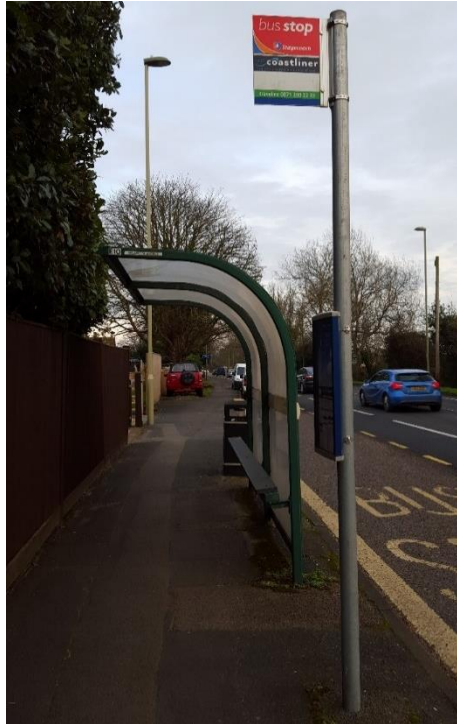
Photograph 7: Havant Road Bus Stop
