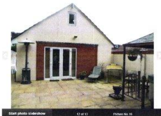
Ancillary accommodation (2011) from private road.
