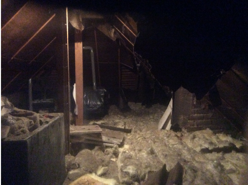
Figure 5. The internal aspects of the roof void at Harbour View.
