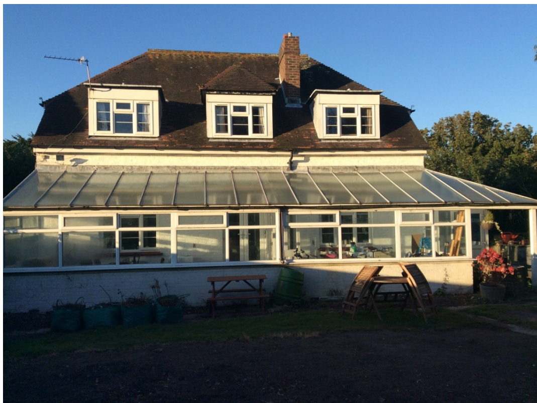
Figure 3. The south facing aspect of the house at Harbour View.
