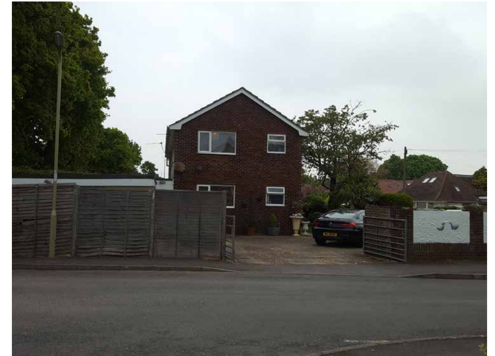
Two-storey house to immediate east of site
