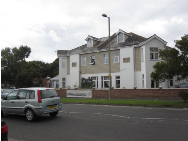
Photograph 3 – showing facade of building, with existing street lighting shown
