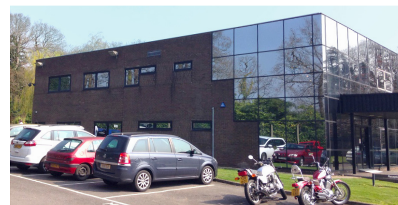
Existing modern office building
