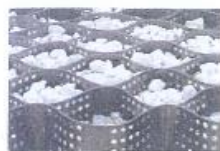
Cellweb TRP across road during filling with green stone.
