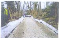
Cellweb TRP across road during filling with green stone.
