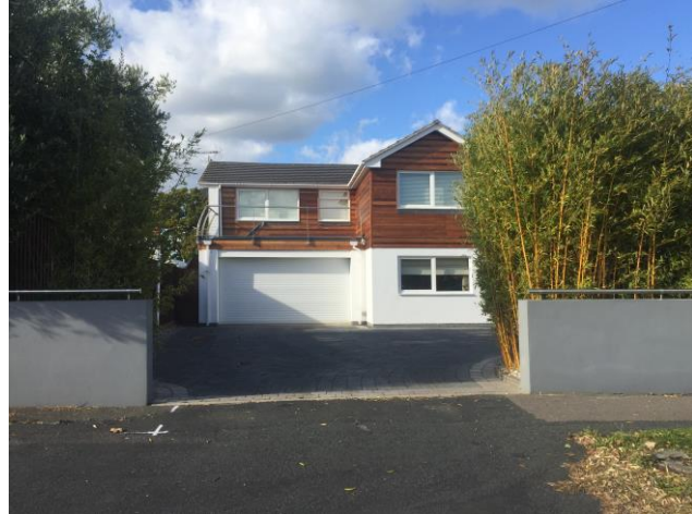
Fig 3: Another dwelling showing two contrasting finishes on the ground and first floor.
