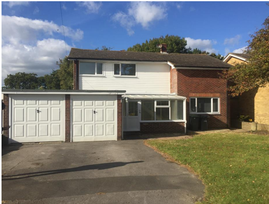
Fig 1, Rear Elevation of Existing Building
