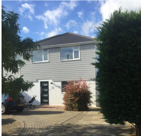
Fig 2: North Shore Road house with white render finish on the ground floor and a timber clad finish on the first floor.
