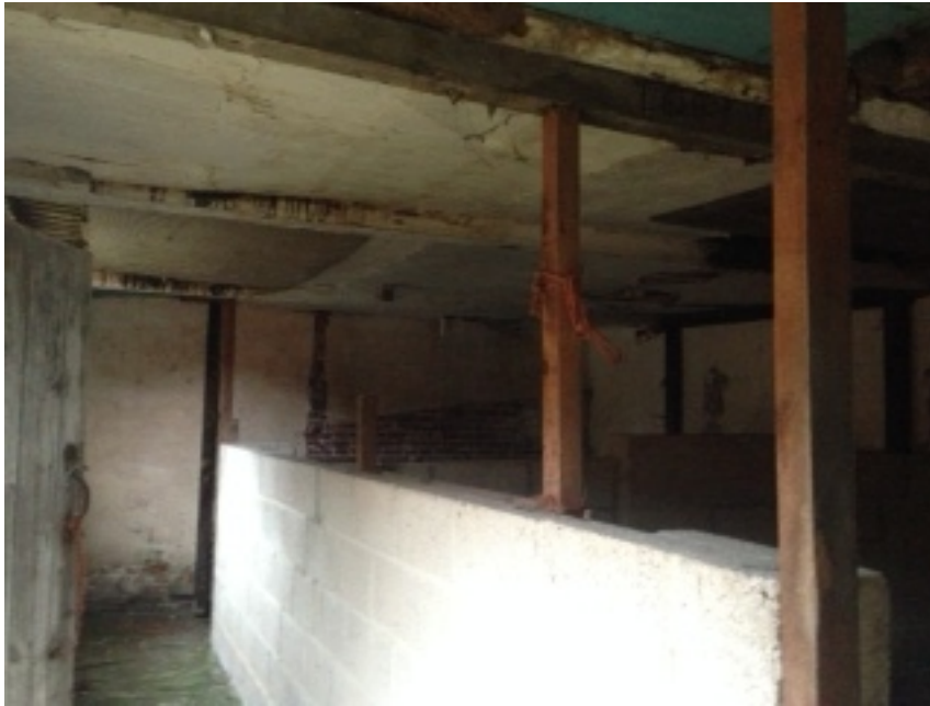
Figure 3. Internal ground level.
