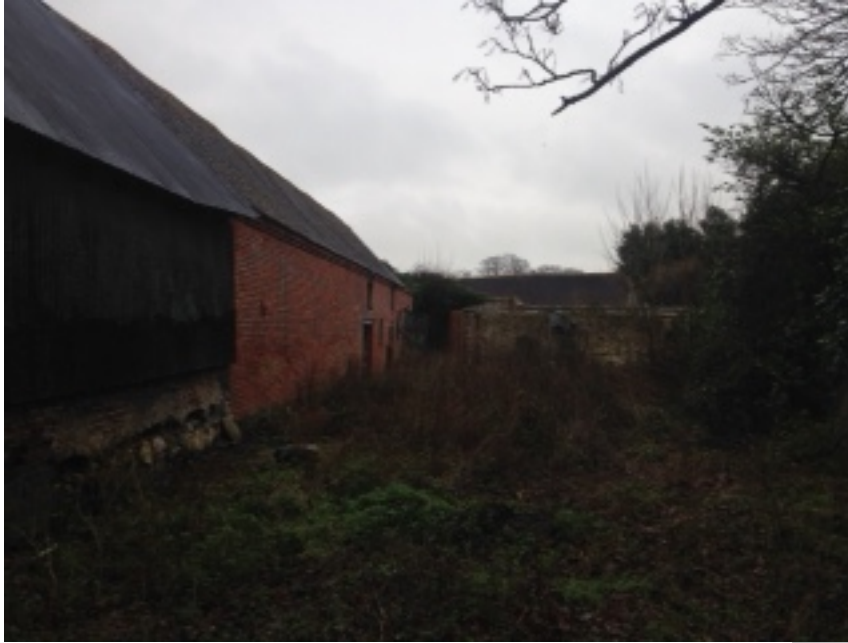
Figure 3. The area of unmanaged grass to the rear of the stable block.
