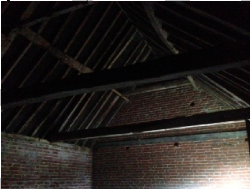
Figure 4. The second storey of the stable block.
