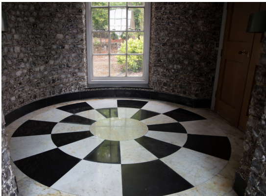
Floor / wall detail
