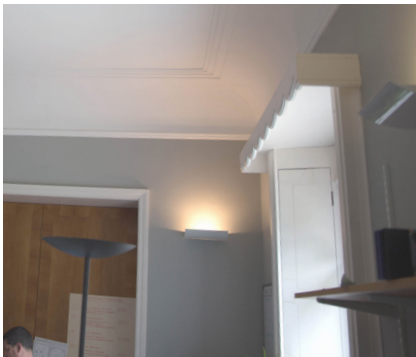
Pelmet / cornice detail
