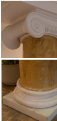
Column & pilaster capital and base
