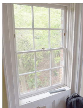
Office F.11 Sash Window
