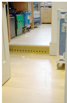
R&D lab timber floor
