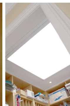
Office F.11 Resource Room ceiling
