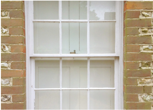
G.07 vertical shutters (viewed from outside)
