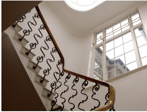
Stairs, landing window and lantern light
