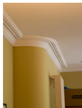
Office F.11 Cornice detail
