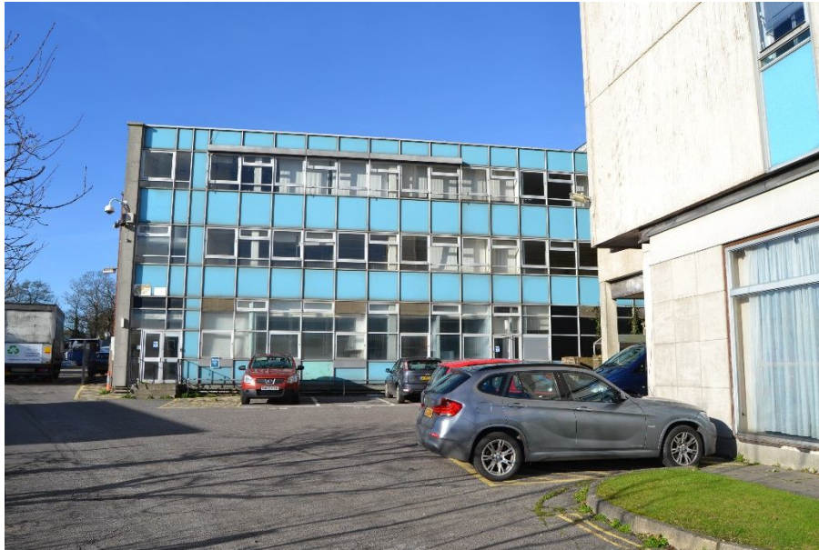
Figure 3: Looking West from New Lane
