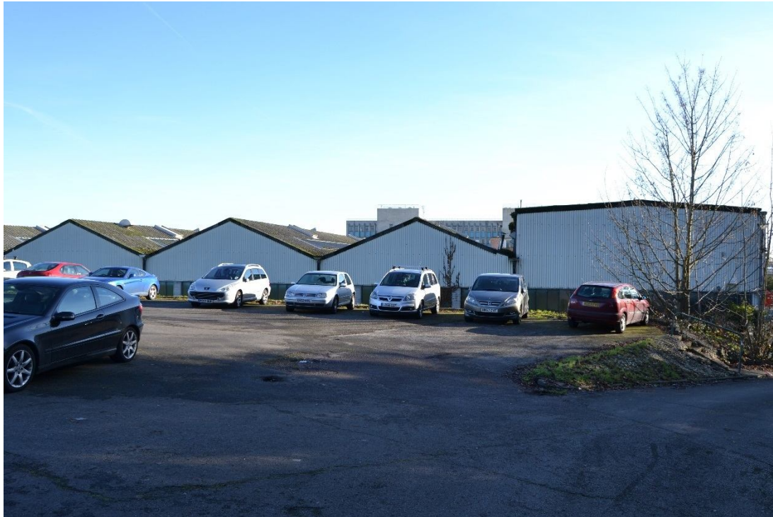
Figure 7: Rear of Site (West Elevation)
