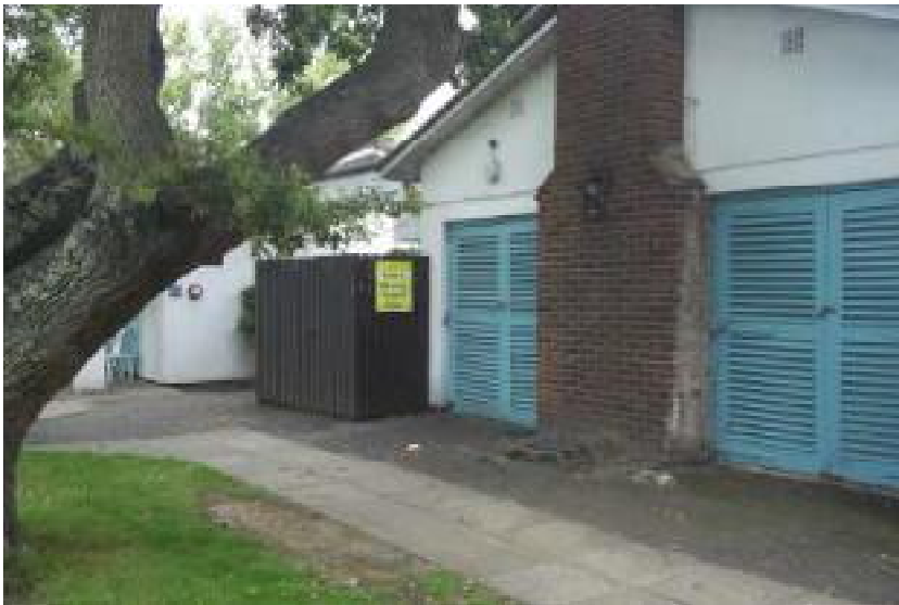
Boiler house and 2x 2500 litre oil tanks in west of site.
