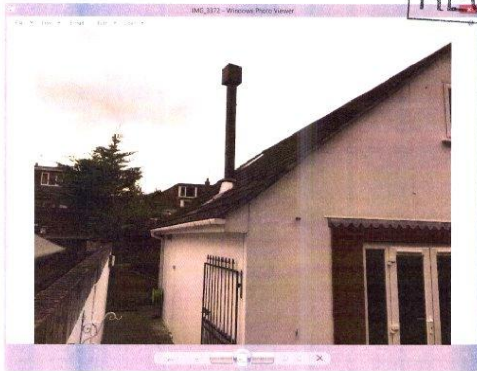
View showing flue exiting roof (Nov 2017)
